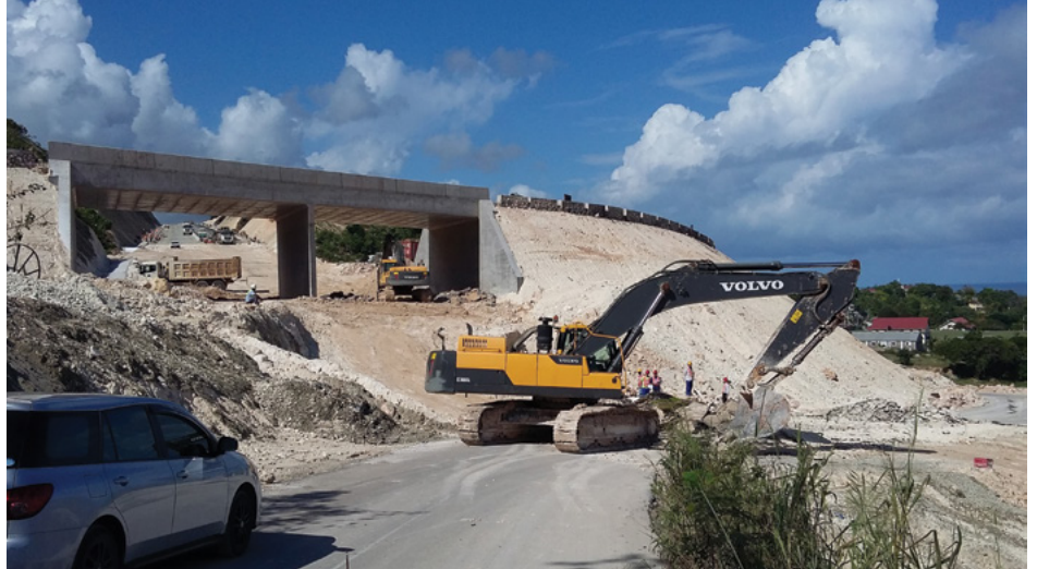
Construction work on the North-South Link of Jamaica's Highway 2000 Project, from Spanish Town to Ocho Rios. The second phase of the Project is a 50-year Concession, held by China Harbour Engineering Company (CHEC).
