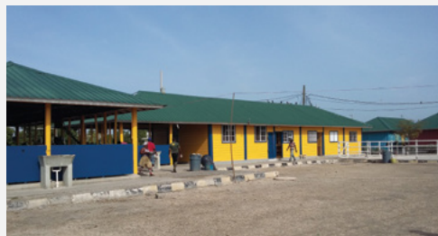
Dyke Road Fishing Complex, Jamaica: Built as part of Highway 2000, to relocate fisher folk who had been illegally occupying lands adjacent to the new Highway, as part of the project’s social responsibility programme.
