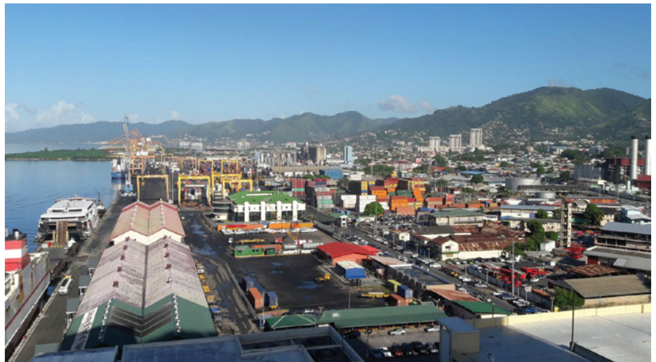
Container Port of Port of Spain, Trinidad and Tobago. PPPs can be used to improve the capacity and efficiency of the Region's ports.
